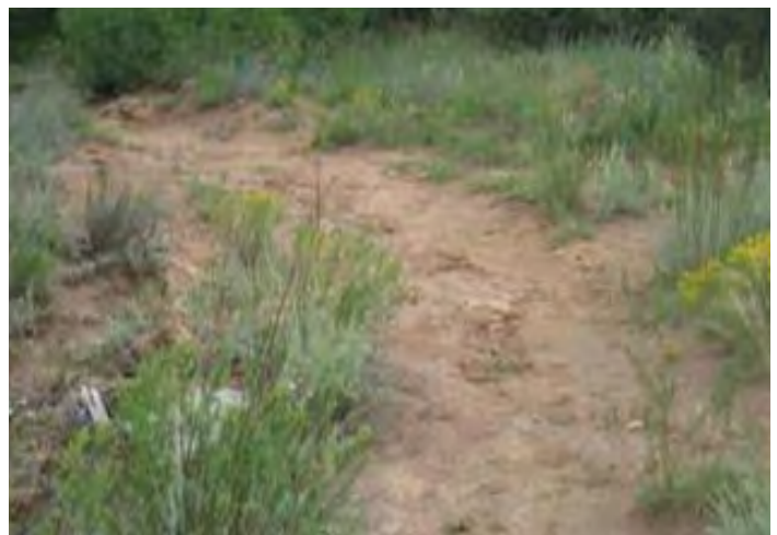
Monitor erosion at trailhead on Barranca Road.
