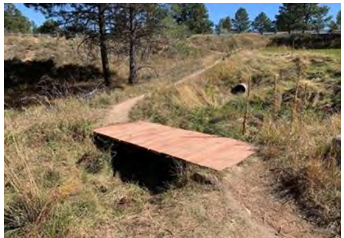
Monitor condition of bridges.
