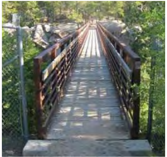
Replace Pueblo Canyon Bridge decking by 2014.
