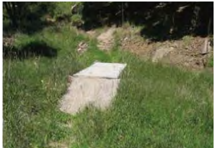
Monitor condition of bridge.
