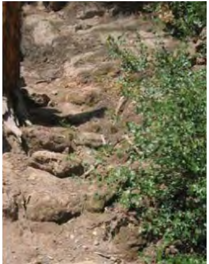
Improve stairs near 34th Street.
