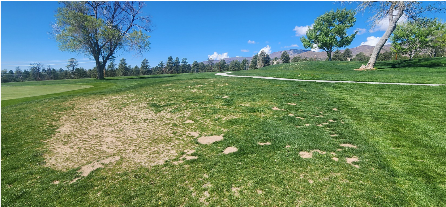
#1 green surround May 3 (old bunker)
