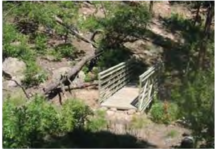
Monitor condition of bridge.
