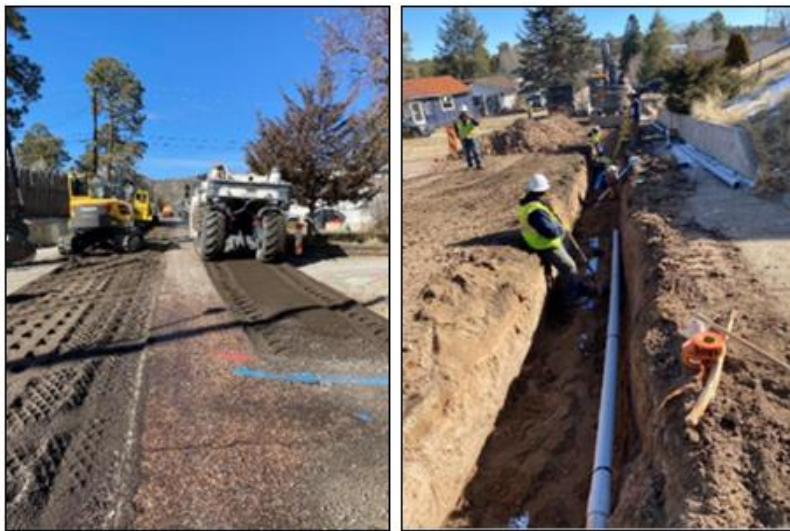
Construction started February 2, 2026, with waterline and broadband installation.
