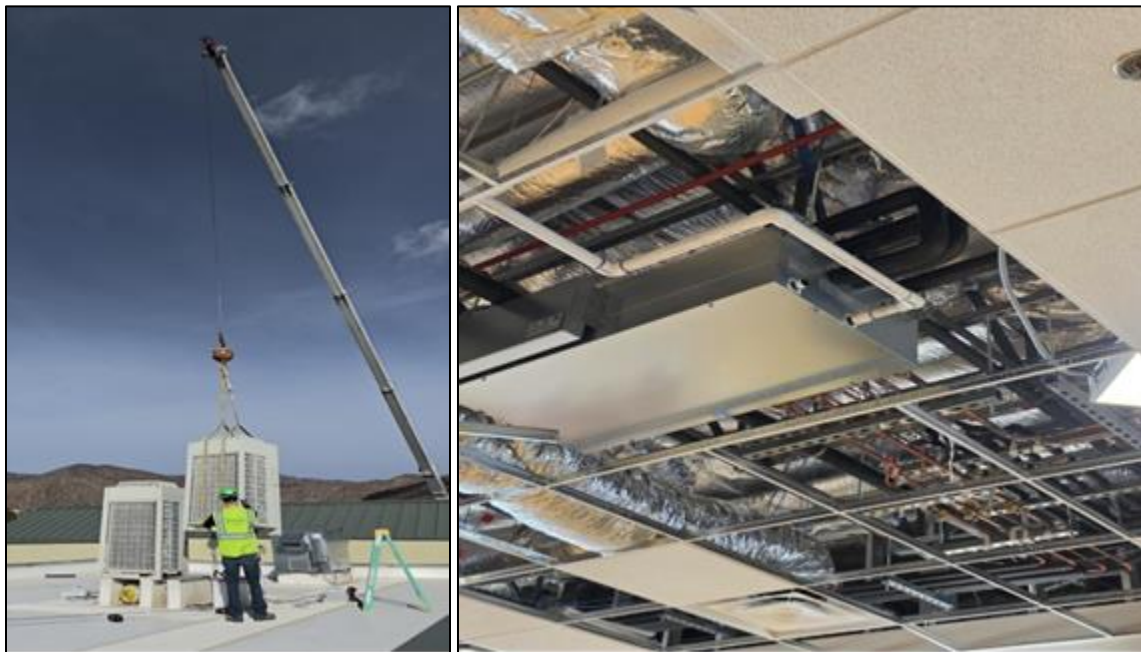
Removal of existing HVAC system and installed new units inside and in the roof of the Clubhouse Community Room.
