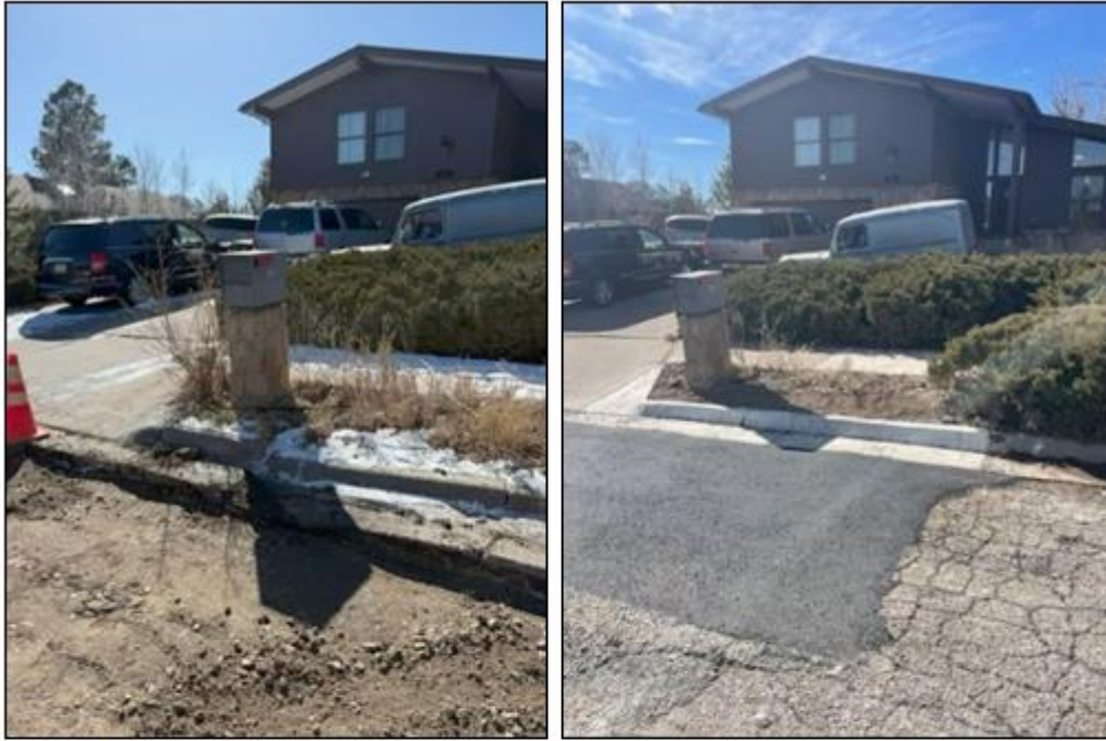
Before and after images of the Streets crew replacing damaged curb on Totavi Street
