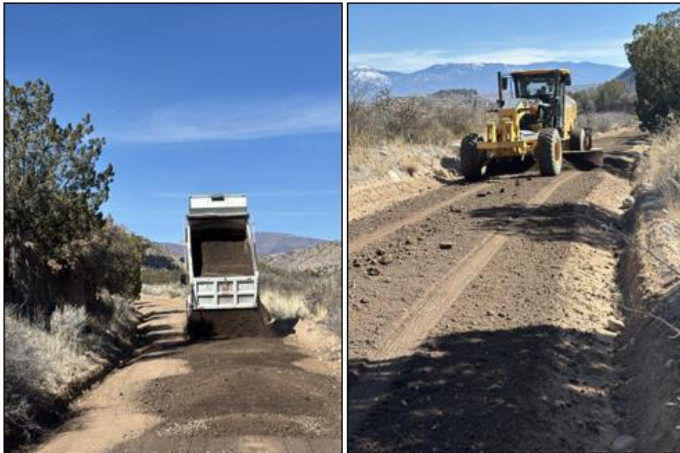
Streets Crews performing Road Maintenance on Rendija Road
