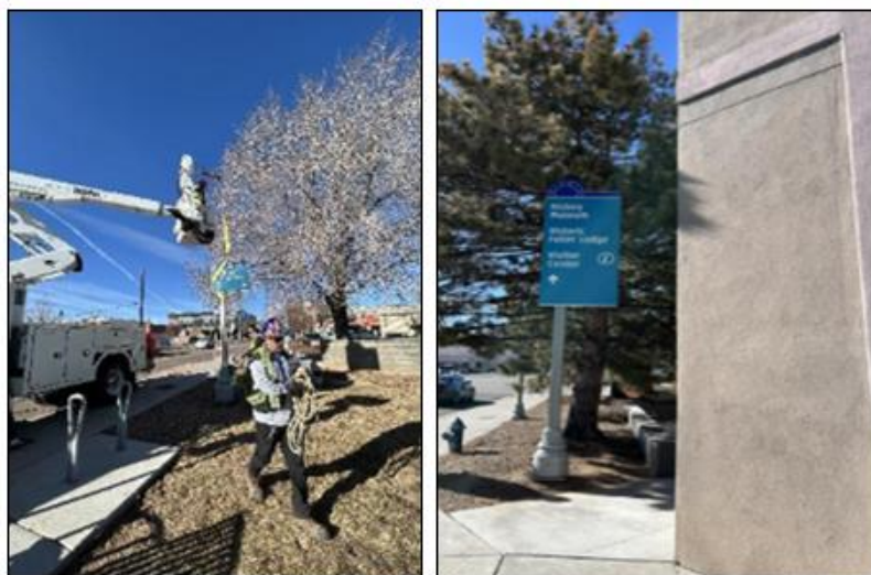
Traffic and Streets crews continue to install wayfinding signs along Central Avenue.
