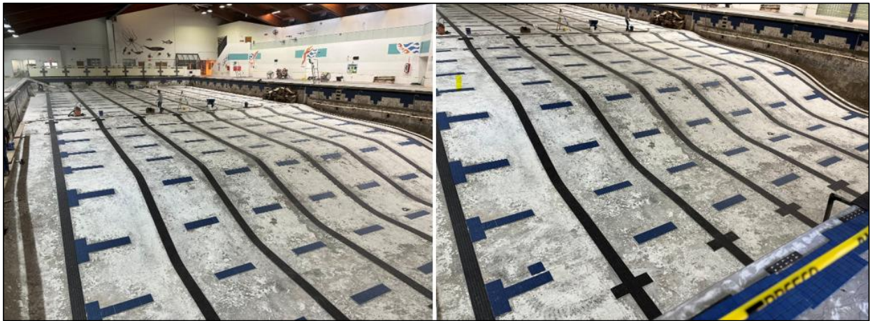
Swim Lane Tile Installation
