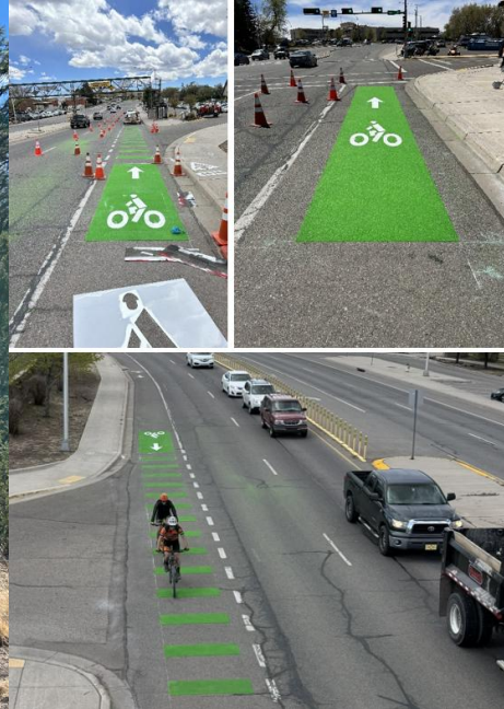
Green Bike Lane Installation
