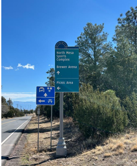
Wayfinding Sign Installation
