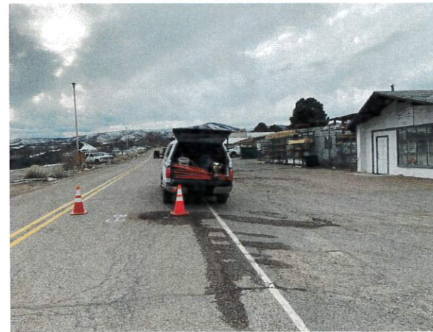
Boring B-3 After Completion
