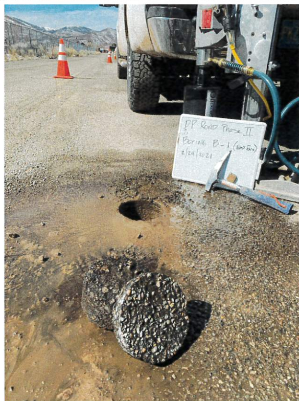
Boring B-1 After Coring
