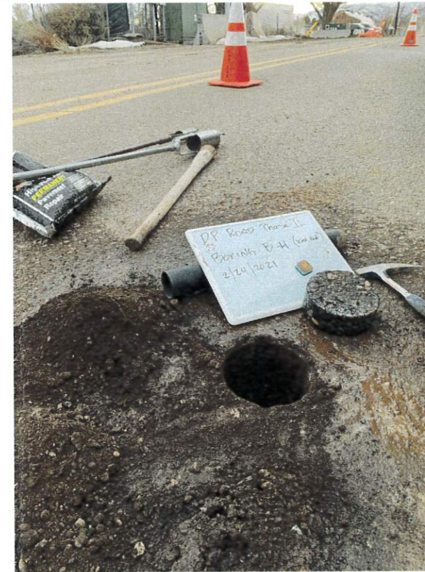
Boring B-4 After Coring
