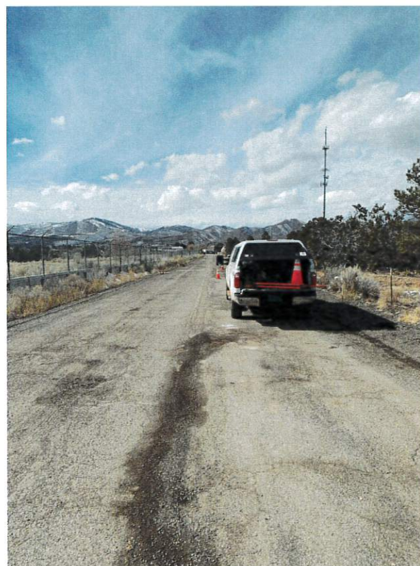
Boring B-1 After Completion
