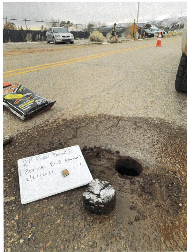
Boring B-3 After Coring
