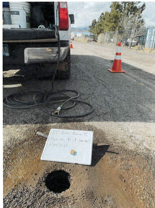
Boring B-2 After Coring
